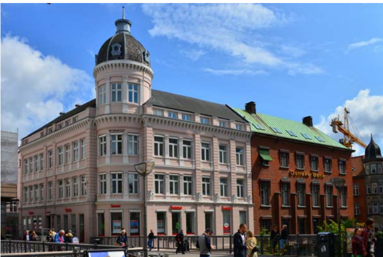
Aarhus Office Building on the Main Pedestrian Street
