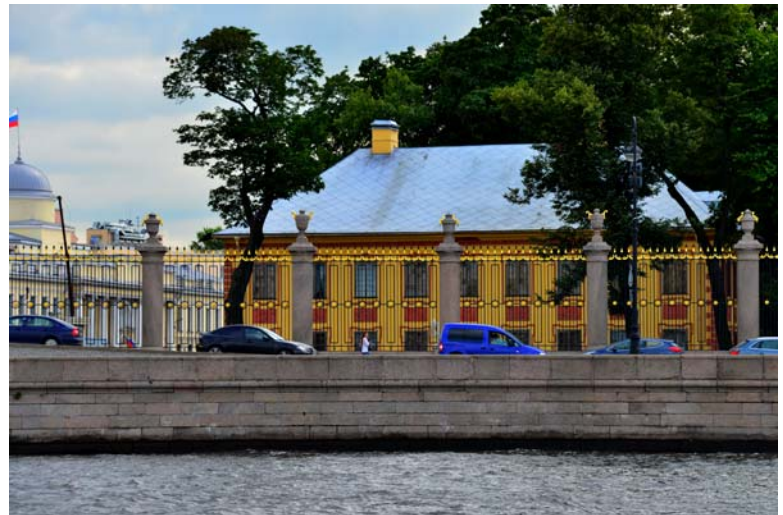
Gold Laced Bldg on Edge of Palace Park
