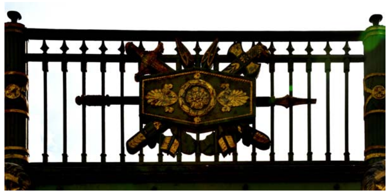
Canal Bridge Railing and Emblem
