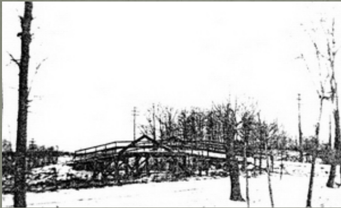
Bushaway Railroad Bridge, 1915
